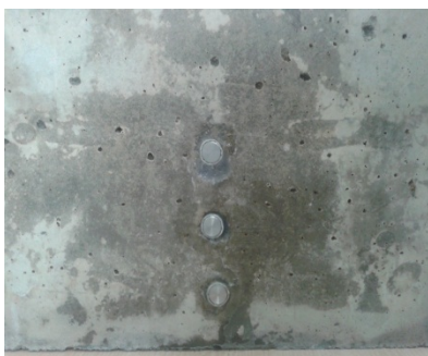
Fig. 11:Mounting water pressure sensors on the dam (reservoir side)
